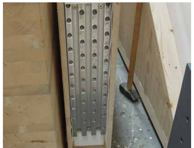
MEGANT® with fire protection Firestrip Interdense Type 15 to protect the connector from heat in case of fire.
