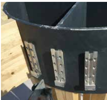
MEGANT® steel connection.
