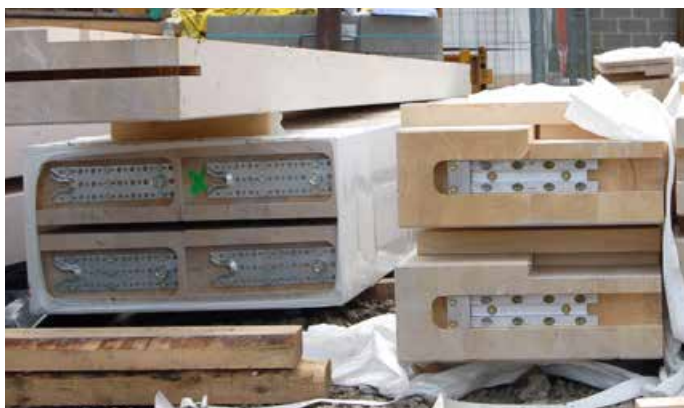
RICON® S milled on three sides in the secondary beam
