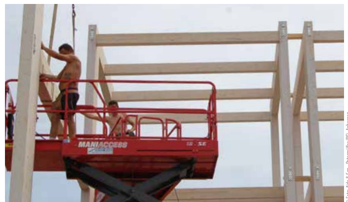
Installation of the secondary support with support by means of RICON® S
