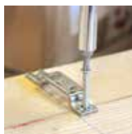
2) Mount KOMBI bracket with screws
