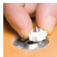
3) Transfer mark with center punch
