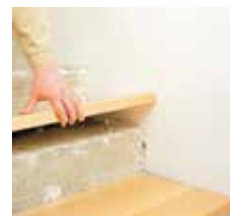
3) Transfer bore holes
