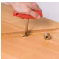
1) Screw-in threaded insert (SW 10)
