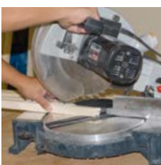
Cut to size glazing bead and FIXclip-profile
