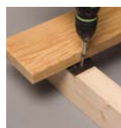
Fasten to the joists with screws
