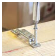
Mount KOMBİ bracket with screws
