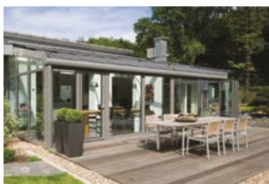
Construction of a sunroom.
