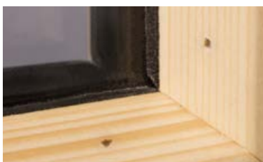
Conventionally fixed glazing bead with visible nails.
