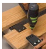
Pre-drill with the template
