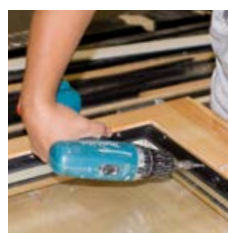
Screw or nail the FIXclip-profile in place
