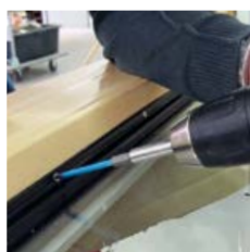
Screw in FIXclip-Profile
