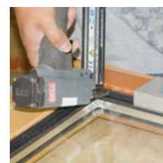
Screw or nail the FIXclip-profile in place
