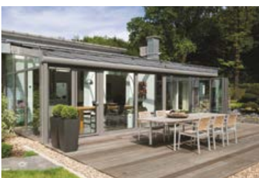
Construction of a sunroom.
