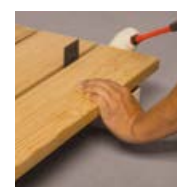
Mount the final board
