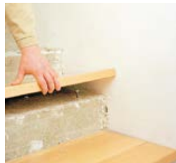
Transfer bore holes
