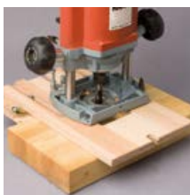
Route mortise with plunge router and routing jig.
