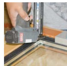
Screw or nail the FIXclip-profile in place
