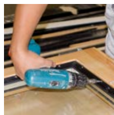
Screw or nail the FIXclip-profile in place
