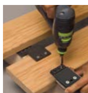
Fasten to the boards with screws
