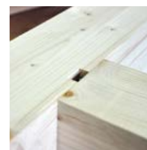
Secured connection using a locking clip
