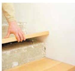
Transfer bore holes
