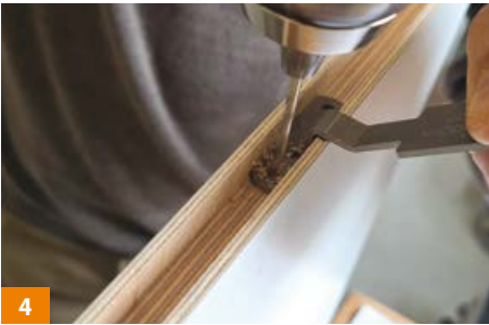
4 Drill the holes using the drilling guide
