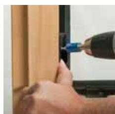
Screw in FIXclip GLE20 in a 45° angle
