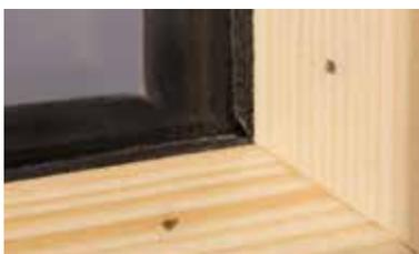
Conventionally fixed glazing bead with visible nails.
