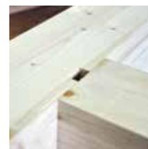
Secured connection using a locking clip
