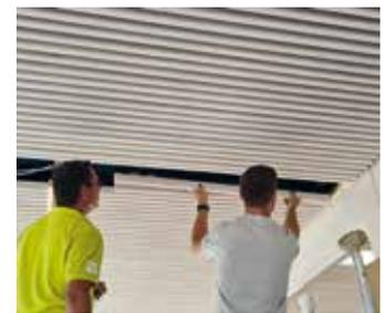
Acoustic ceiling, training room, Knapp GmbH (Austria) | Design in white glazed fir with DEKCLICK® clamp connector.
