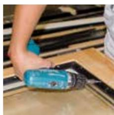
Screw or nail the FIXclip-profile in place
