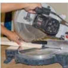
Cut to size glazing bead and FIXclip-profile
