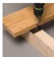
Fasten to the joists
