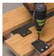
Fasten to the boards with screws
