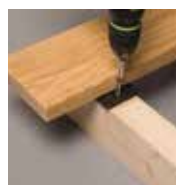
Fasten to the joists with screws
