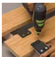
Pre-drill with the template
