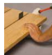
Mount the final board
