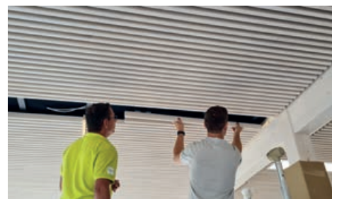
Acoustic ceiling, training room, Knapp GmbH (Austria) | Design in white glazed fir with DEKCLICK clamp connector and beam with MEGANT® connector.
