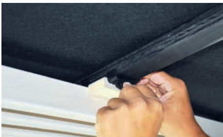
Acoustic ceiling, training room, Knapp GmbH (Austria) | Design in white glazed fir with DEKCLICK clamp connector and beam with MEGANT® connector.
