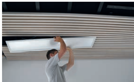
Acoustic ceiling, training room, Knapp GmbH (Austria) | Design in white glazed fir with DEKCLICK clamp connector and beam with MEGANT® connector.
