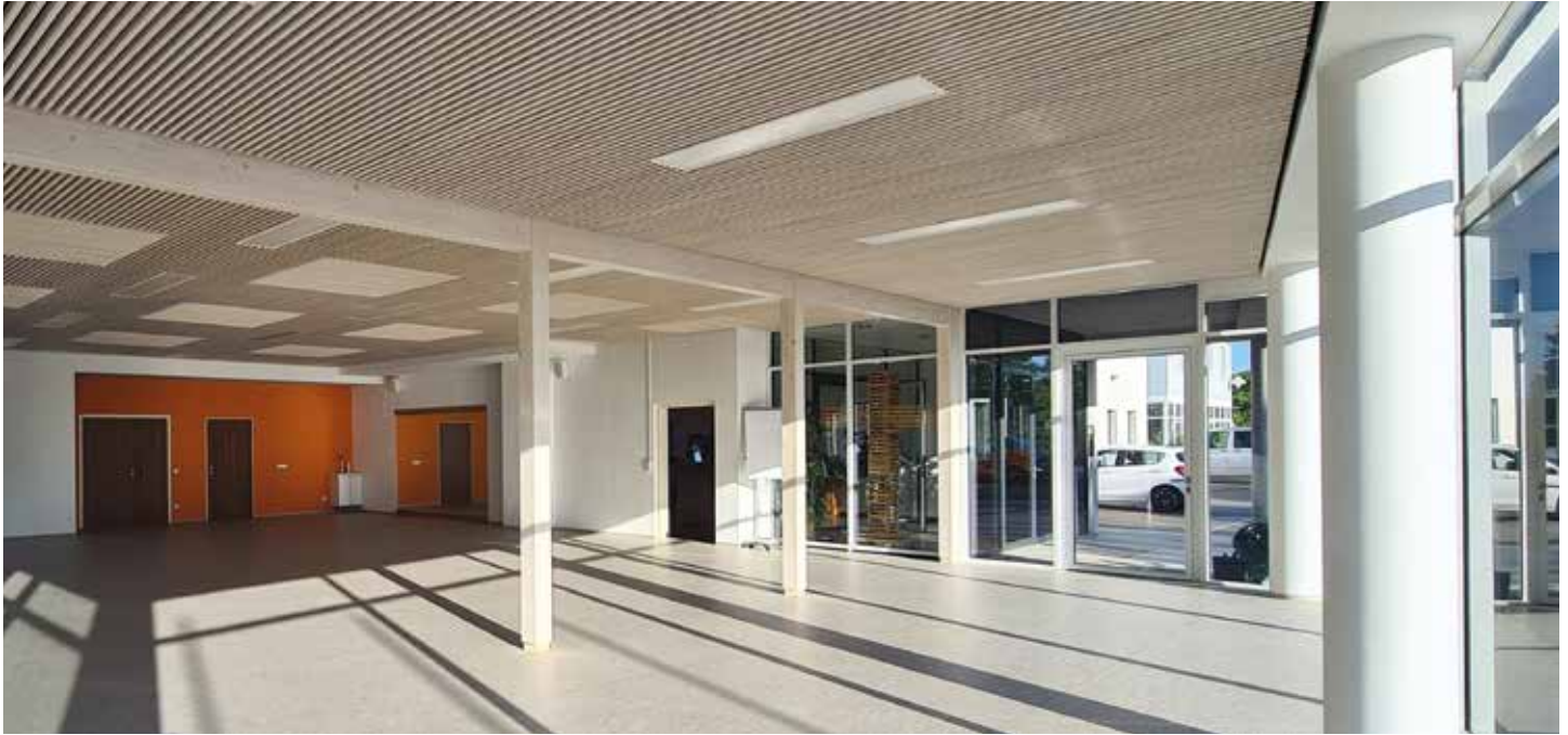
Acoustic ceiling, training room, Knapp GmbH (Austria) | Design in white glazed fir with DEKCLICK clamp connector and beam with MEGANT® connector.
