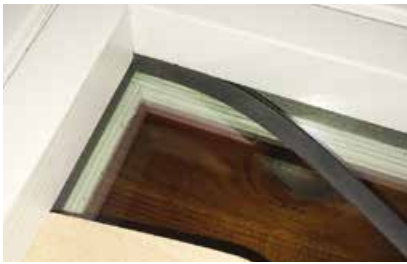
Example: Mounting wedge-shaped sealing
