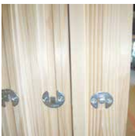
Instruction example: Mounting of window elements with DUO30
