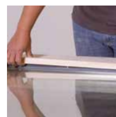
4) Clip on glazing bead.
