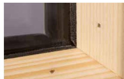
Unsightly attaching of glazing bead with nails.
