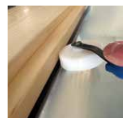
5) Clean finish with sealing roller
