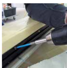
2) Fix FIXclip-Profile with nail/screw
