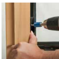
1) Install FIXclip GLE20 Plus in screw in 45° angle
