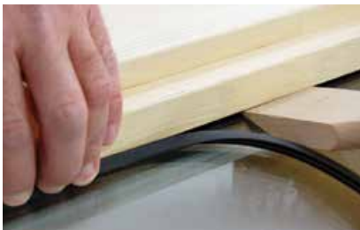
Press in wedge-shaped sealing
