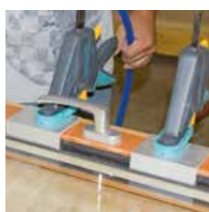
2) Pressing pane of glass against outer seal
