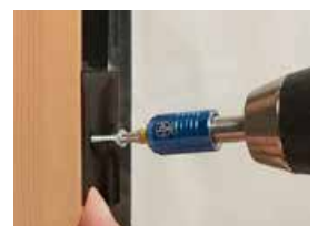
Continued applied pressure due to fixing with screw in 45°
