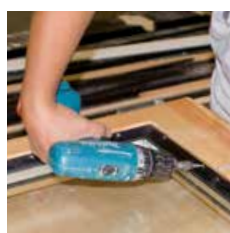
3) Screwing or nailing the FIXclip-Profile
