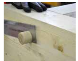
Cut off the excess sand smooth.
