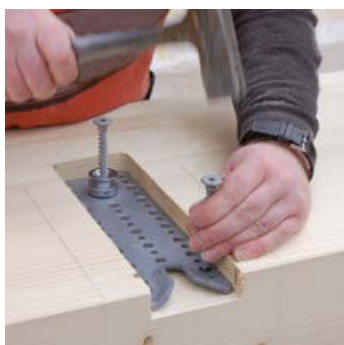
Position the plate and the screws
