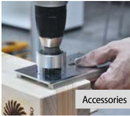
Manual processing with KNAPP® drilling templates.
