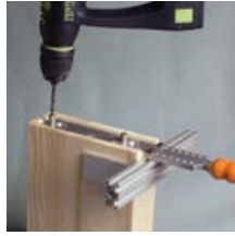
Pre-drill with drilling-jig
