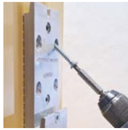
3. Screw the second plate onto the secondary beam.
