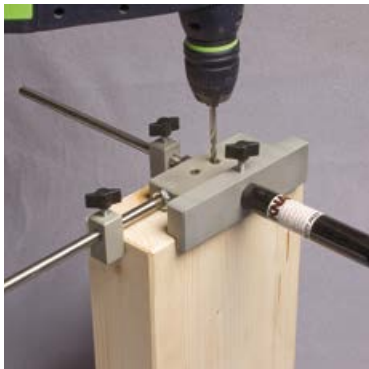
Pre-drill secondary beam
