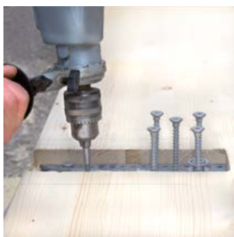
Screw on RICON®S on Header
