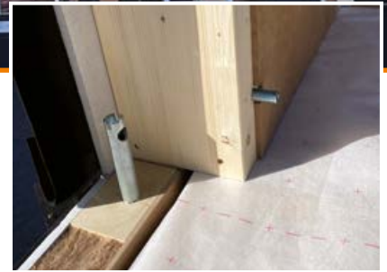
Installation example: Wall to wall connection with Pipe System.
