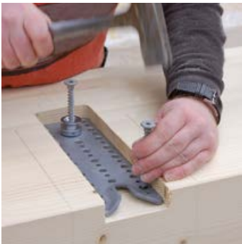
Position the plate and the screws
