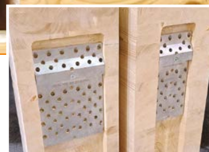
Installation example: Standard version, bolted on
