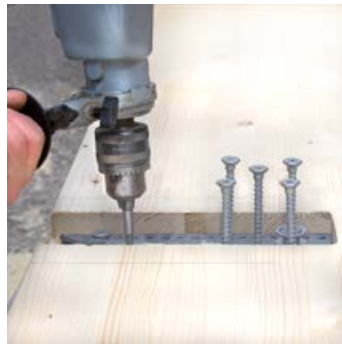
Screw on RICON®S on Header
