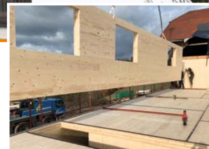
Installation example: CLT walls installation.
