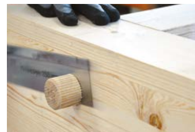
Cut and sand the excess part
