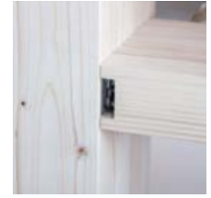
Secure connection with locking clip
