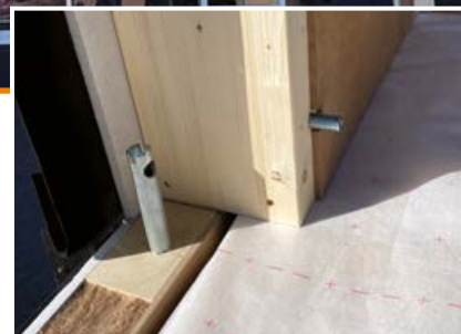
Installation example : Wall to wall connection with Pipe System.
