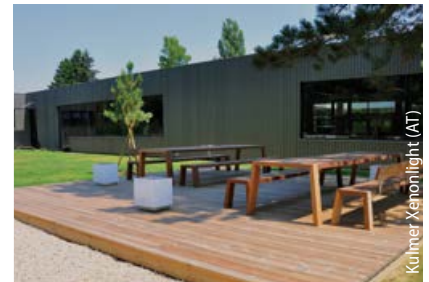
Terrace built with QUATRO 65
