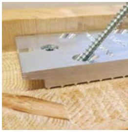
2. Screw in the horizontal screws, then screw in the diagonal screws..
