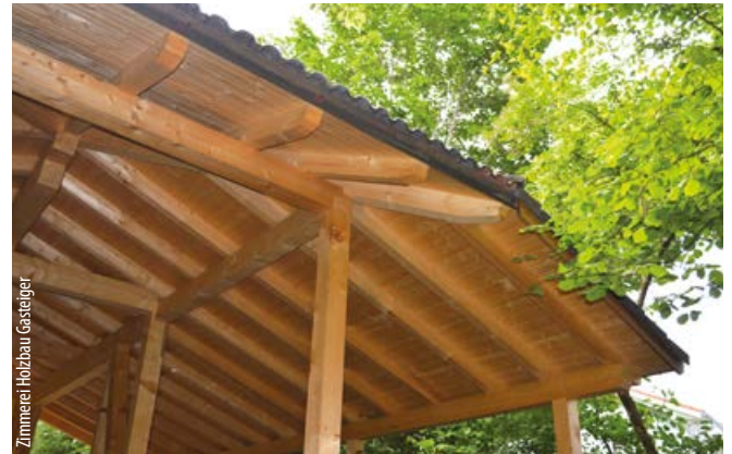
Carport without brace.
