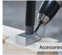
Pre-drill at an angle using the KNAPP® drilling template.
