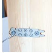
Install the locking clip
