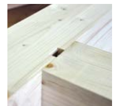
Secured connection using a locking clip
